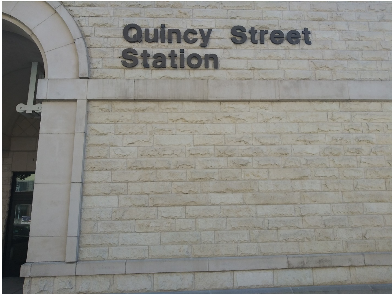
Outdoor Picture 5 West Wall South of Quincy Street Entrance
